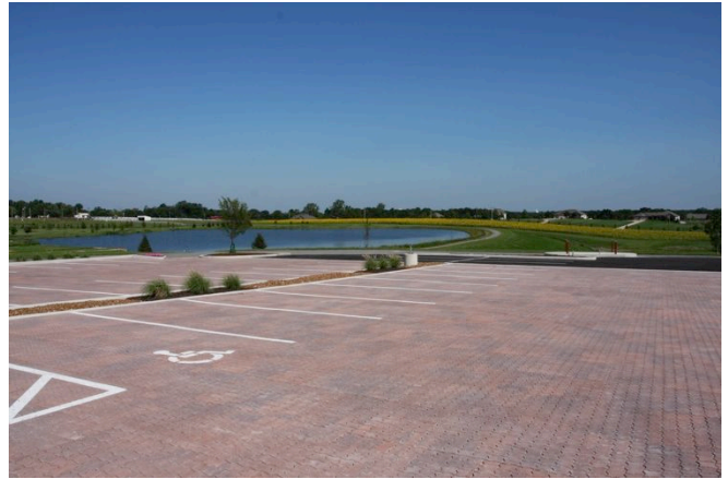
Example of permeable paver parking at the Jefferson Farm.
